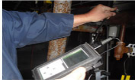
NDT Ultrasonic Thickness Measurements
